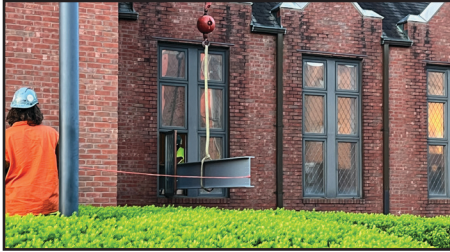
The steel beam to support the choir loft was lifted via crane, brought in through a window, and installed along the back wall of the chapel.
