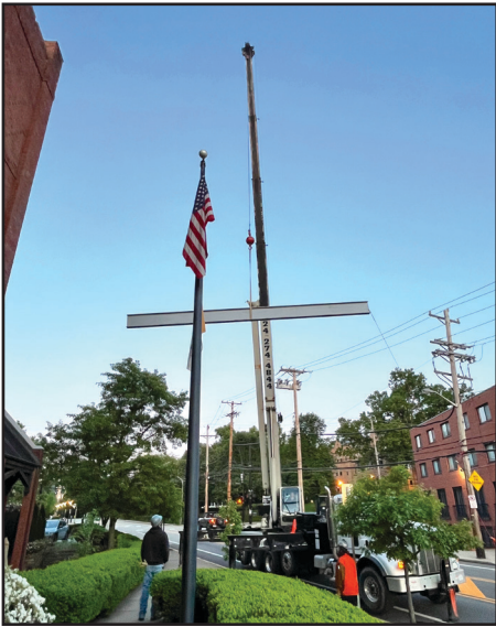
The steel beam to support the choir loft was lifted via crane, brought in through a window, and installed along the back wall of the chapel.
