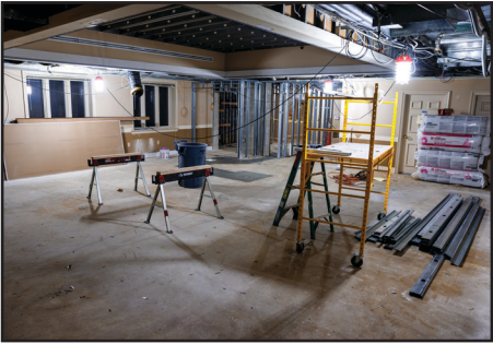
Old lighting, well-worn carpeting and aged ceiling tiles removed from student center in preparation for replacement.
