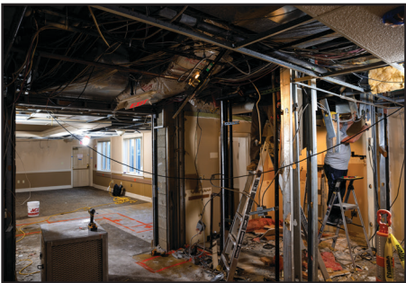
Demolition of the downstairs Student Center:
